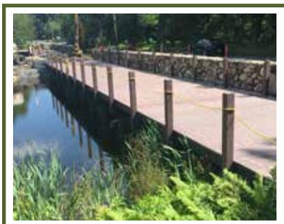
NOTE: Spacing between intermediate rails/pickets is set at 3-3/4" (max). In order to comply with International Building Code (IBC) requirement that a 4" sphere shall not be allowed to pass through openings.
